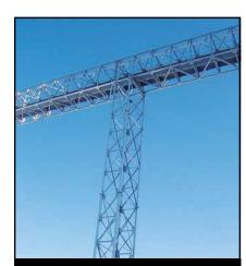
Catwalk Support Towers are custom engineered for height, wind, speed or seismic zone. Freestanding or guyed, with the option to add access bracing, conveyors, spouting and other custom configurations.
