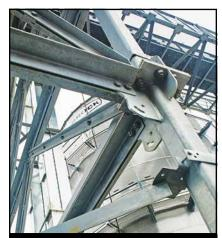
**Slot & Tab System** is precision fabricated for exceptional column strength.
