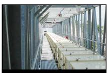
Walk-Through Truss comes in standard widths of 72-120 inches (1828-3048 mm) and maximum span of 190 feet (57.9 m). Custom engineered spans can reach up to 270 feet (82 m) and longer.
