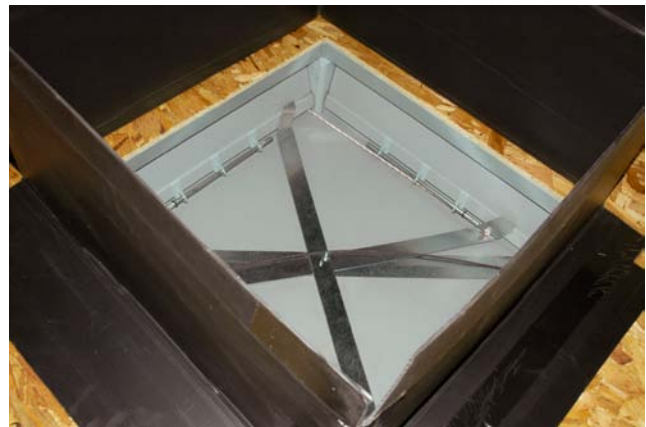
Top view of inlet from the attic in closed/locked position.
